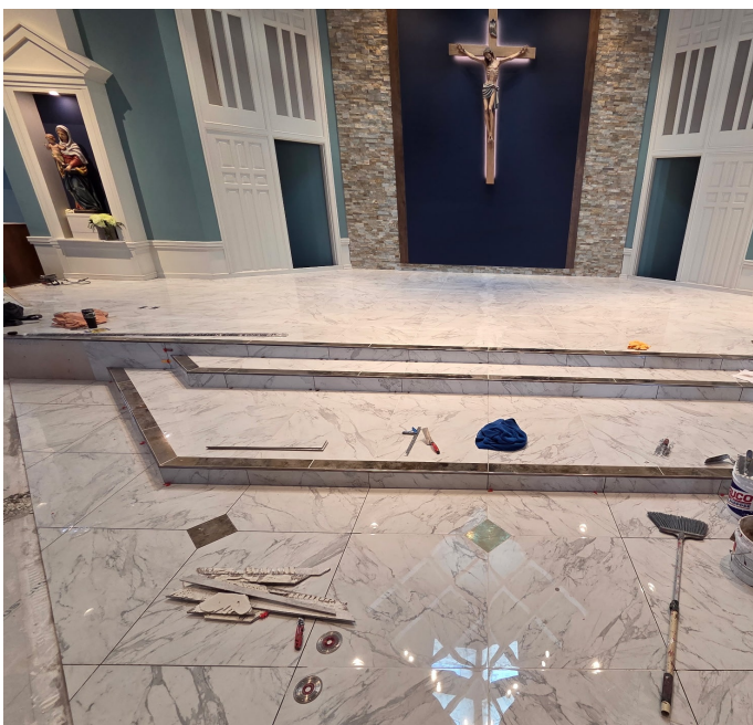
St. Philip Catholic Church | Franklin, TN Sanctuary tile High-quality finish installation
